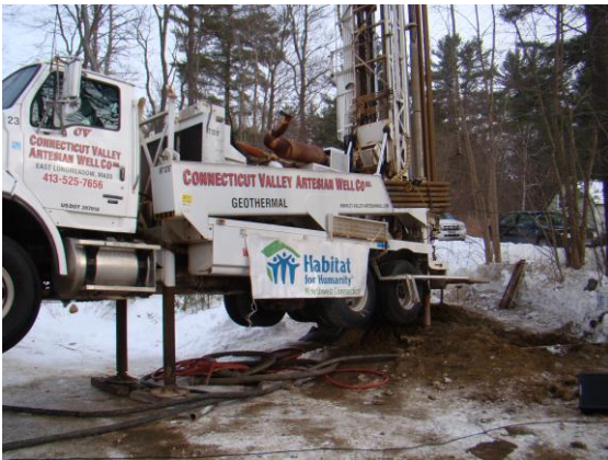
Start of borehole drilling by CT Valley Artesian Well Co, Inc.
